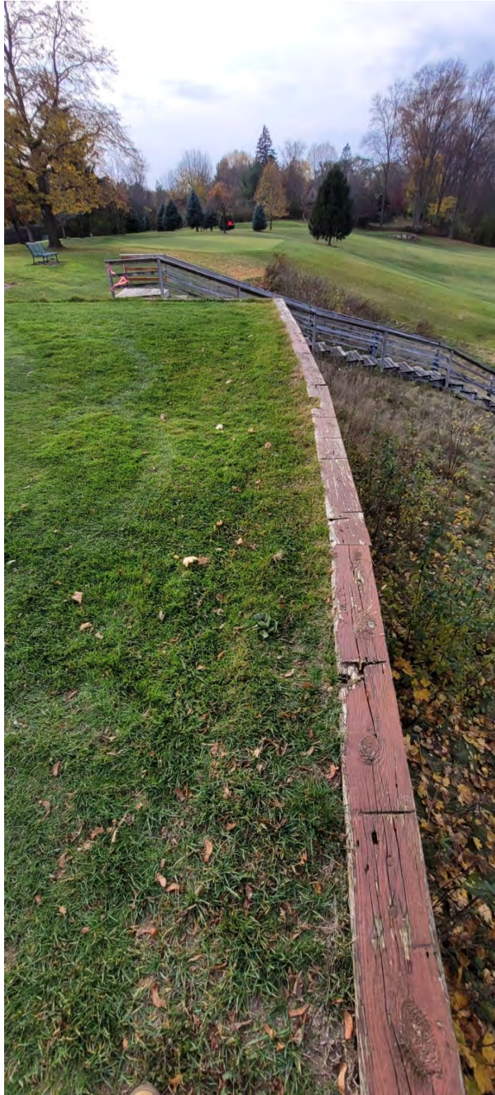
View West from Tee towards Staircase
